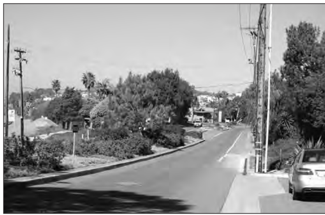
The inconvenience of driving in and out of Del Mar along this stretch of Jimmy Durante Boulevard should come to an end in about a month. Street, sidewalk and drainage improvements that started in February are expected to wind down by May 24. Photo by Bianca Kaplanek
